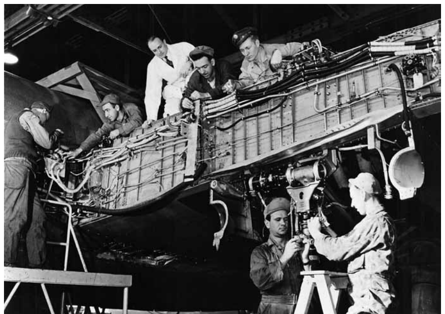
Electrical mechanics-in-training work on the miles of wiring in a B-29's wing spar. Because of new and revolutionary materials and features incorporated, the workers faced a steep learning curve.
